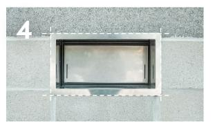
**Check Flange Frame Placement** Ensure flange frame is level, flush with the wall, and firmly adhered.
