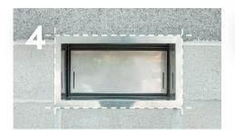
Check Flange Frame Placement Make sure flange frame is level, flush with the wall, and firmly adhered.
