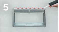
Apply Sealant on Fire Damper Apply fire barrier along all 4 sides of the fire damper.
