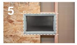
Check Frame Placement Make sure the vent frame is level and flush with the wall.
